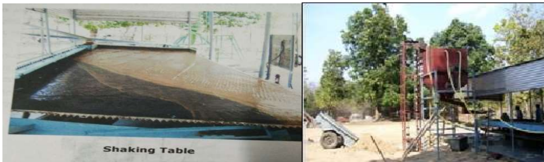
Treatment of Raw Sand and Siri River Unit
